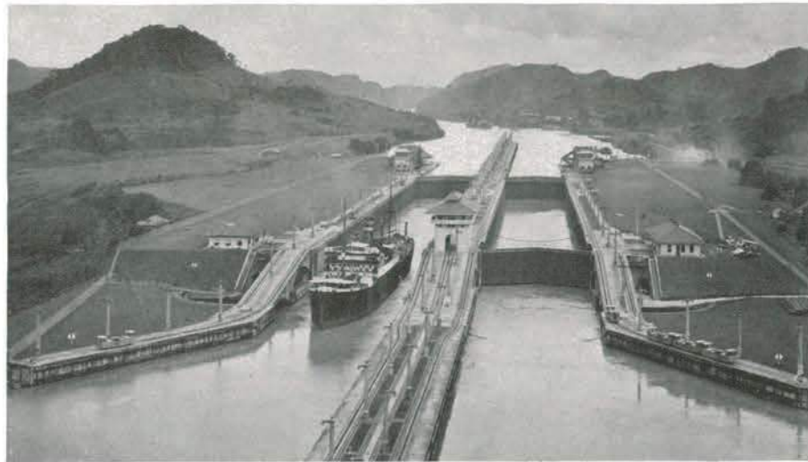
View of the present double set of Pedro Miguel locks with Gaillard Cut in the distance, Lake Miraflores in the foreground.
