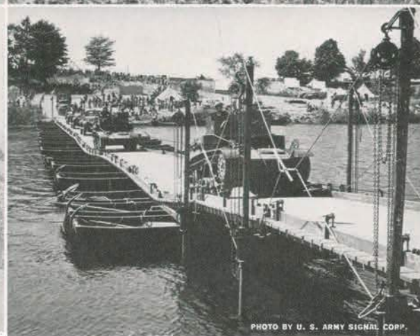
Rushed to a river, a pontoon train quickly throws across a bridge that will support the heaviest mechanized units.
